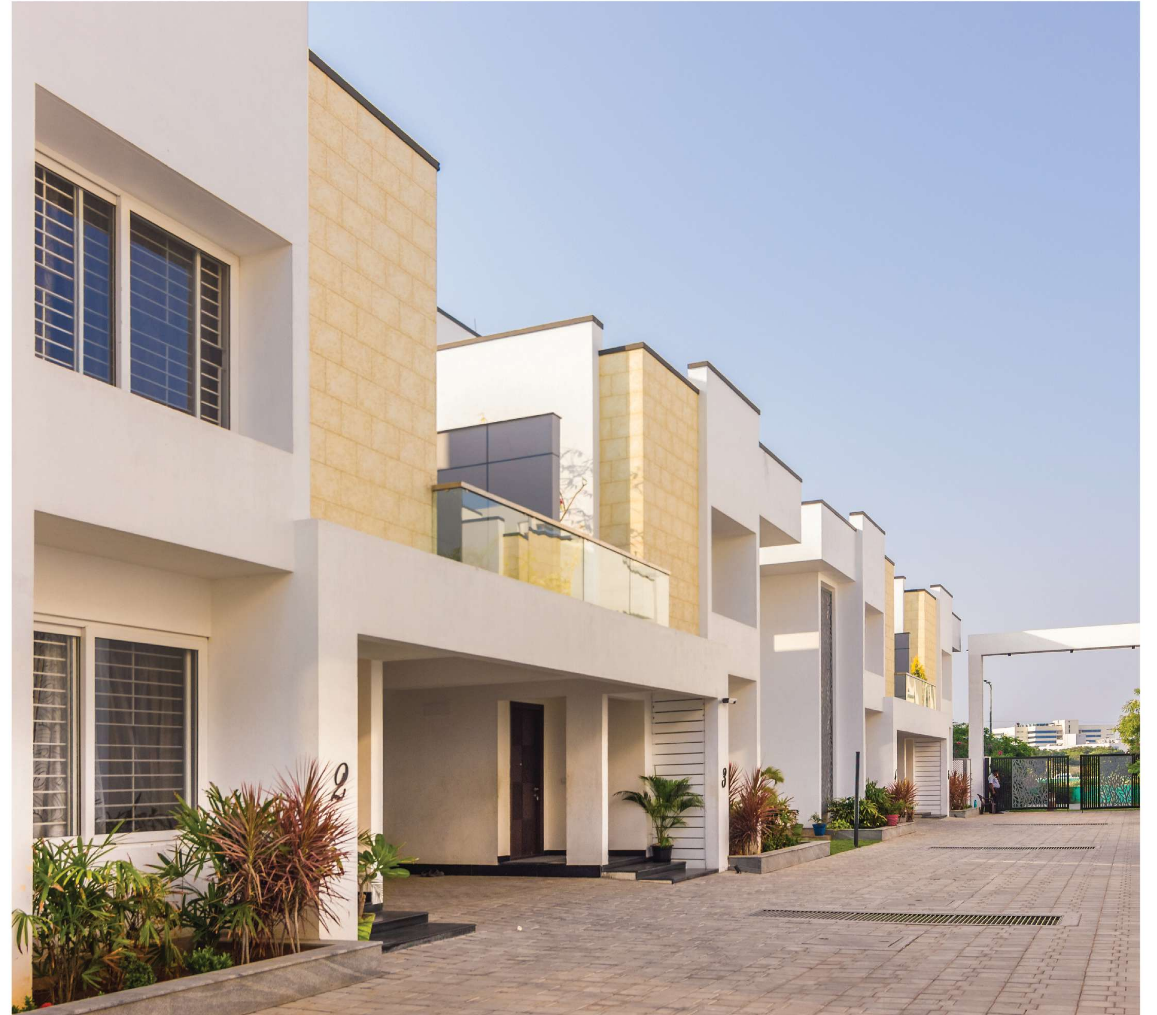
Insignia, Perungudi (Architect: Pramod Balakrishnan)
