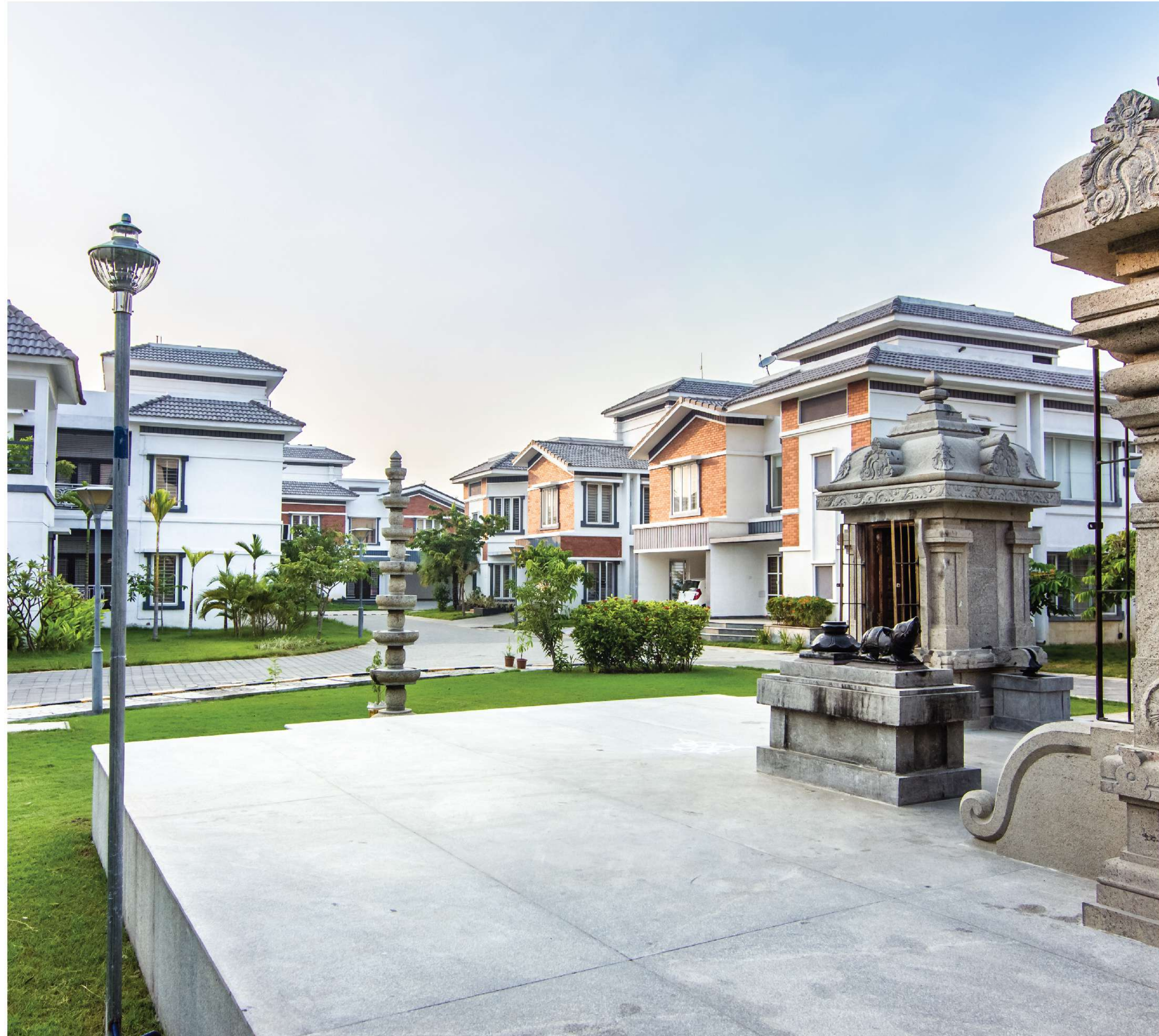
Villa Padmalaya, Karapakkam (Architect: Transform Design)
