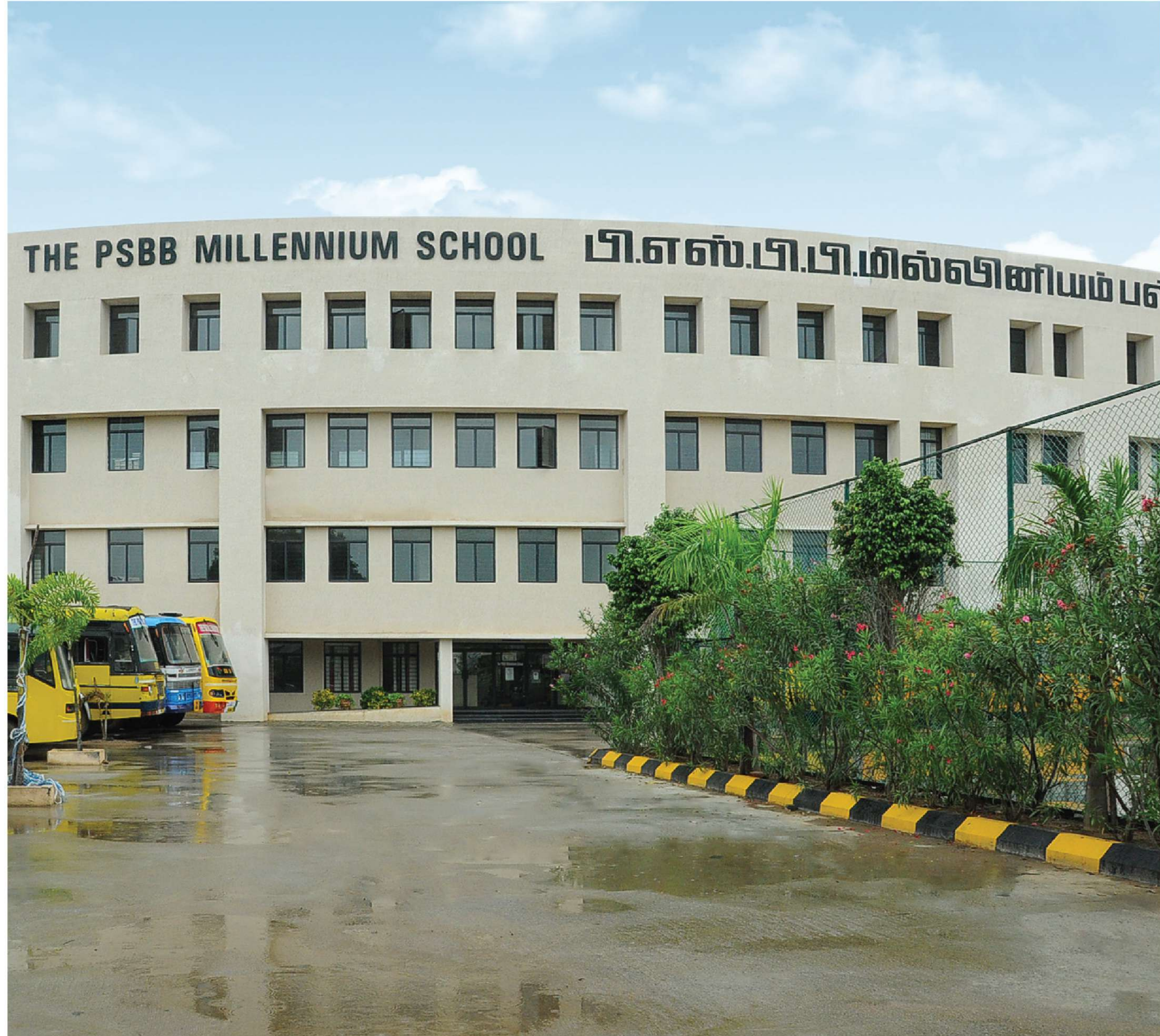
The PSBB Millennium School, Gerugambakkam (Architect: Vijay Gupta Architects, Delhi)
