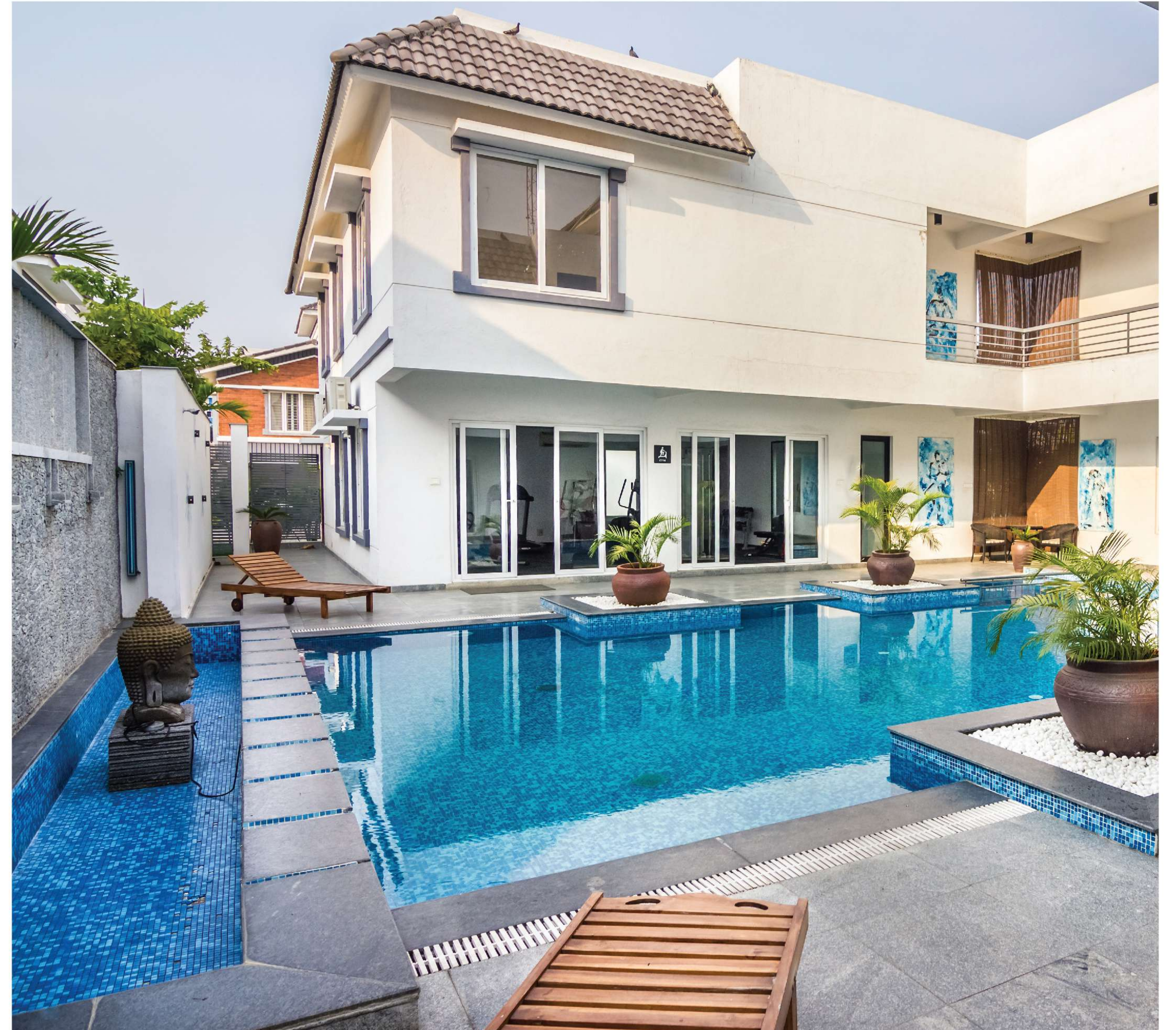
Villa Padmalaya, Karapakkam (Architect: Transform Design)
